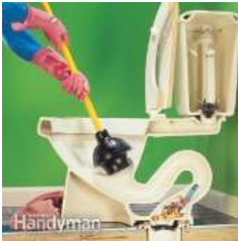
Fig1: fixing a clogged toilet with rubber plunger retrieved from http://www.familyhandyman.com/plumbing/toilet-repair/how-to-fix-a-clogged-toilet/view-all
